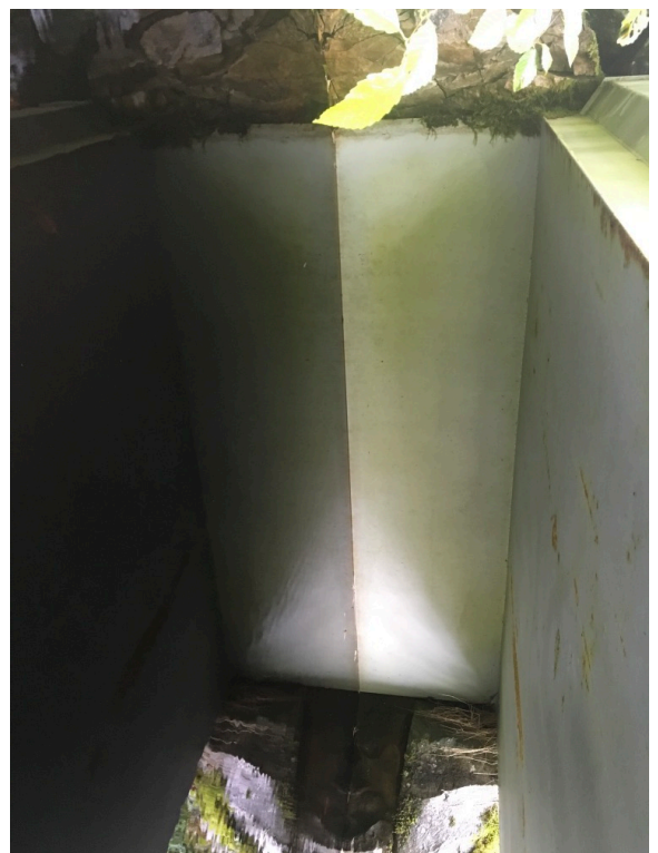
Left Bank Abutment when facing downstream
